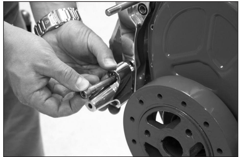
Figure 4: Install Tensioner Support Bracket
